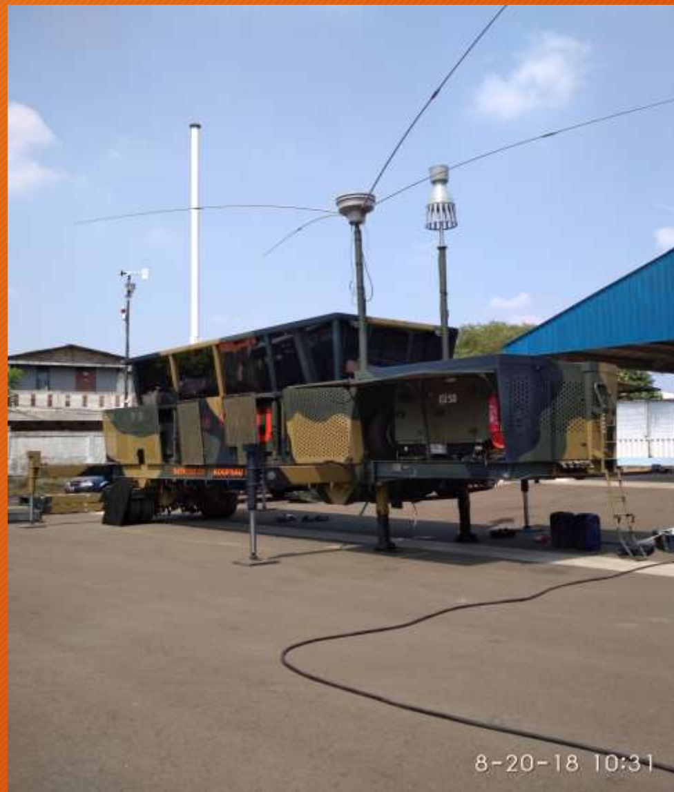
Pekerjaan Repair ATC Tower mobile TA.2018
